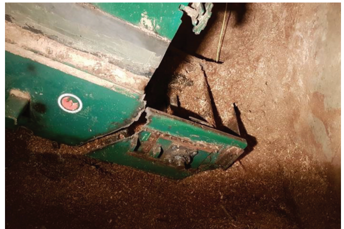
Guard was removed and not replaced on the conveyor
