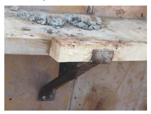
Having reviewed the manufacturer's instruction for use, it was noted that at least one manufacturer did not allow "walers brackets" to be used as scaffold brackets. They were to be used only to straighten the form walls and not as a work platform, as doing so would contravene paragraph 9(2)(a) of the Occupational Health and Safety Act, which states:
